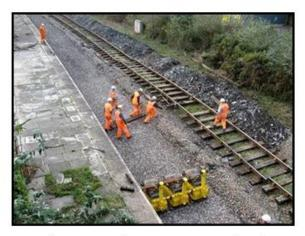
3. Sleepers needing repair were replaced, &
